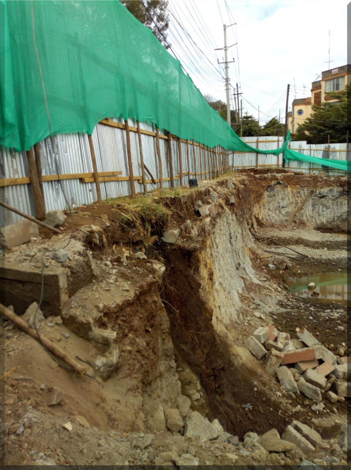
Fig. 04. Excavation works in progress
