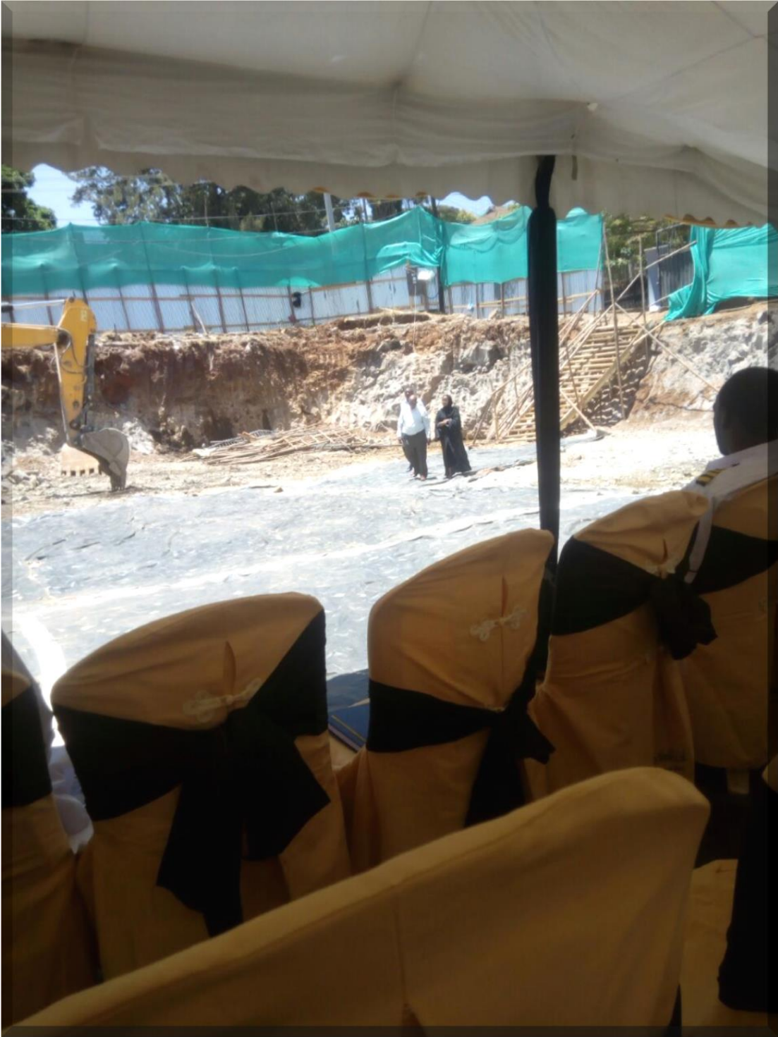
Fig. 03. Excavations almost complete waiting trimming as below
