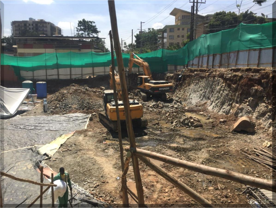
Fig. 05. Excavations works progressing on as below
